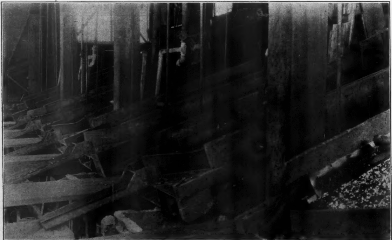
The Vibrating Screens
